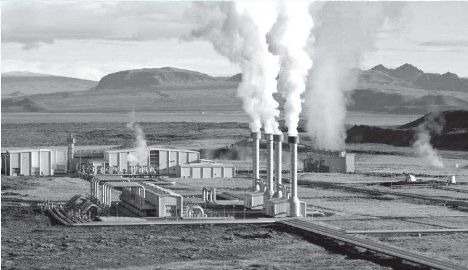
Nesjavellir geothermal power station, Iceland. Due to the high concentration of volcanoes, Iceland has an unusual advantage of utilizing geothermal energy. Shown here is Nesjavellir Geothermal Power Station with a capacity of 120 MW.
